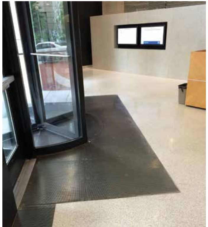
The George Washington School of Public Health in Washington, D.C., provides walk-off mats to control dirt and dust. (Sara Hamerschmidt)
