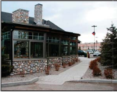
Direct and visible walkway link between parking and retail space -West Market Square, Calgary
