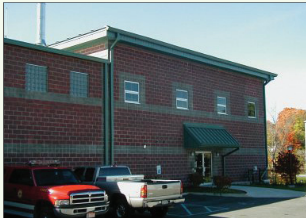
Northern Westchester Joint Water Works Filtration Plant (Town of Cortlandt) 2
