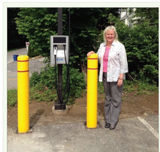
Supervisor Linda D. Puglisi in Front of the EV Charging Stations Installed at Town Hall in 2014 (Dani Glaser)
