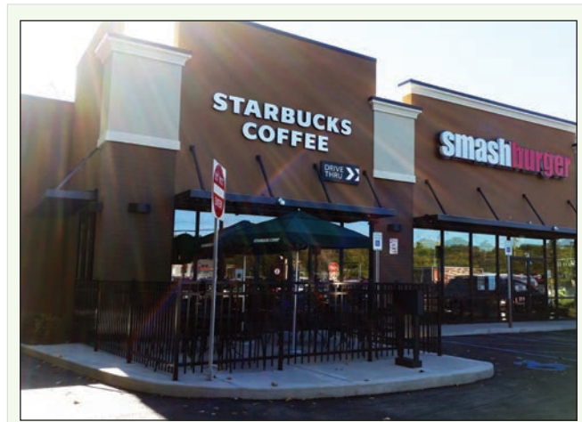
Recent Commercial Development along Route 6 (Town of Cortlandt)
