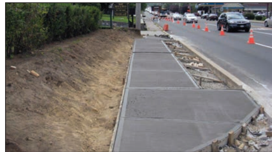
Ongoing Pedestrian Improvements to Cortlandt Boulevard (Town of Cortlandt)
