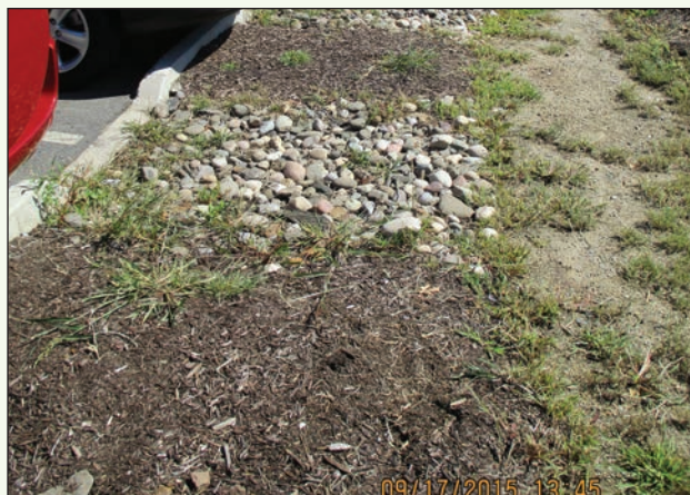
Stormwater Swales along Route 6 (AKRF, Inc.)
