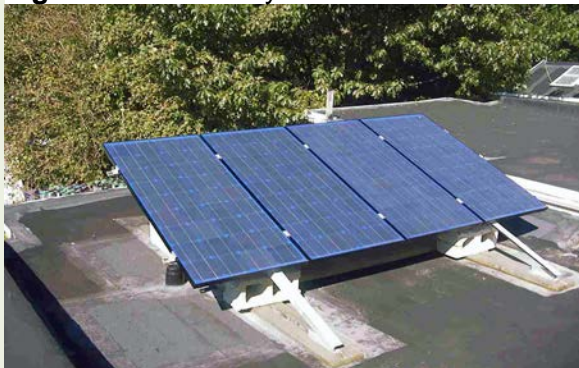
Figure 6: A Tilted System on a Flat Roof
