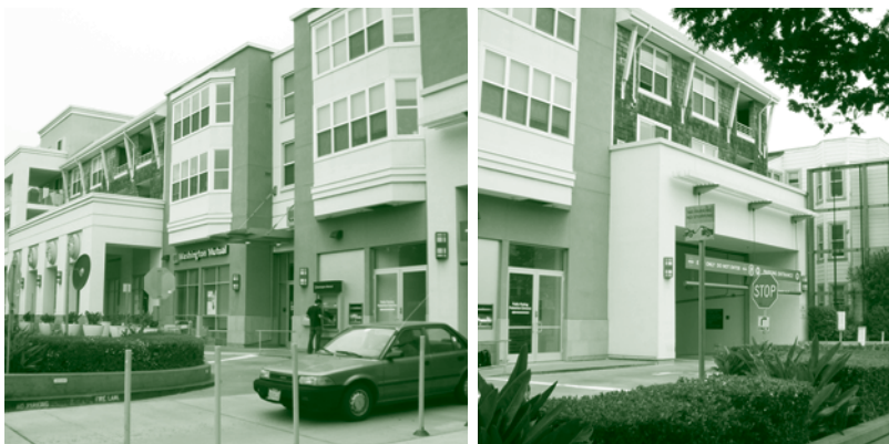
From left to right: Grocery storefront, Retail (bank), parking entrance
