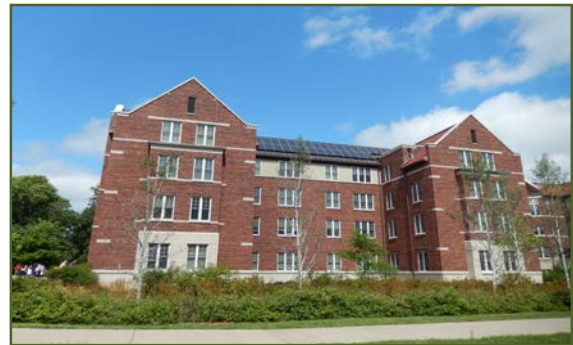
Rooftop Solar, CERTs
