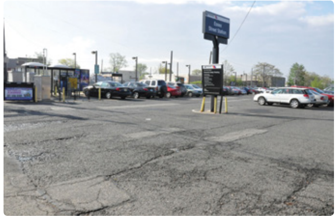
Figure 71: View of existing Essex Street commuter parking lot
