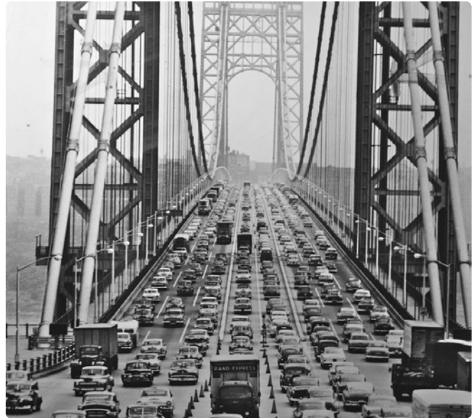
Figure 29: George Washington Bridge connecting Bergen County and NYC
