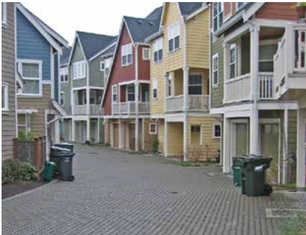
Permeable pavers in High Point, Seattle, WA Source: Brett VA, Creative Commons
