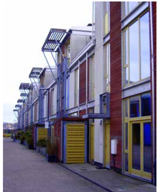
Live work units in North Greenwich, London Source: European Institute for Sustainable Transport, Creative Commons
