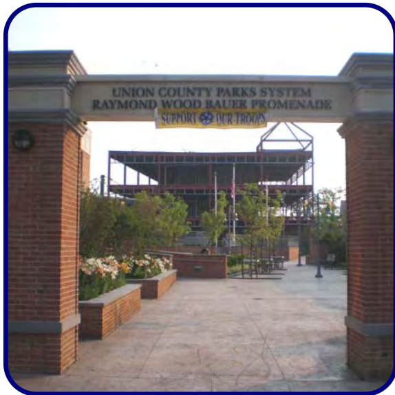
The Raymond Wood Bauer Promenade and the building under construction are results of the Theater Site Redevelopment Plan.
