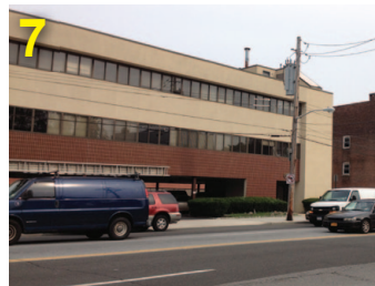
7 Poor quality storefront
