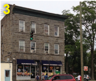
Attractive brick facades
