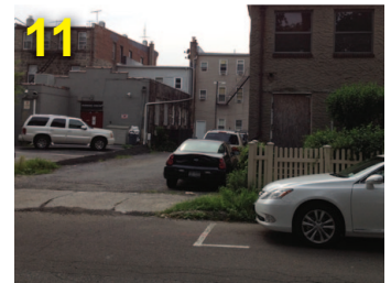
11 Rear entrances in poor condition
