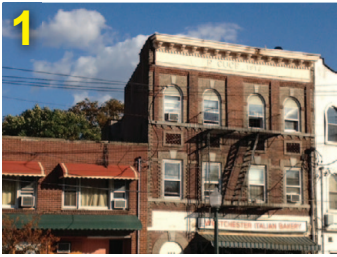
Attractive brick facades
