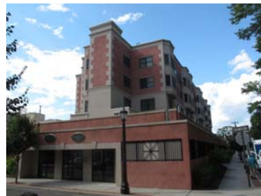
Ground-floor parking allows for flooding with minimal damage. All residential uses located on higher floors.
