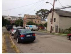
Buildings/sidewalk in disrepair
