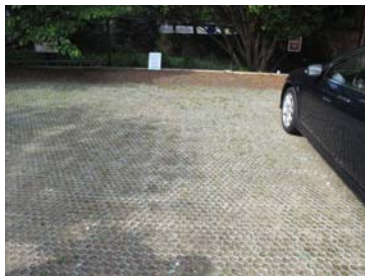
Use of permeable pavement to reduce stormwater runoff
