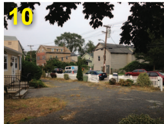
10 Yard in poor condition
