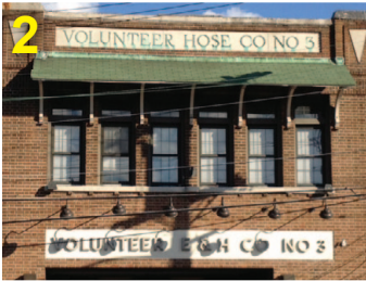
Attractive brick facades
