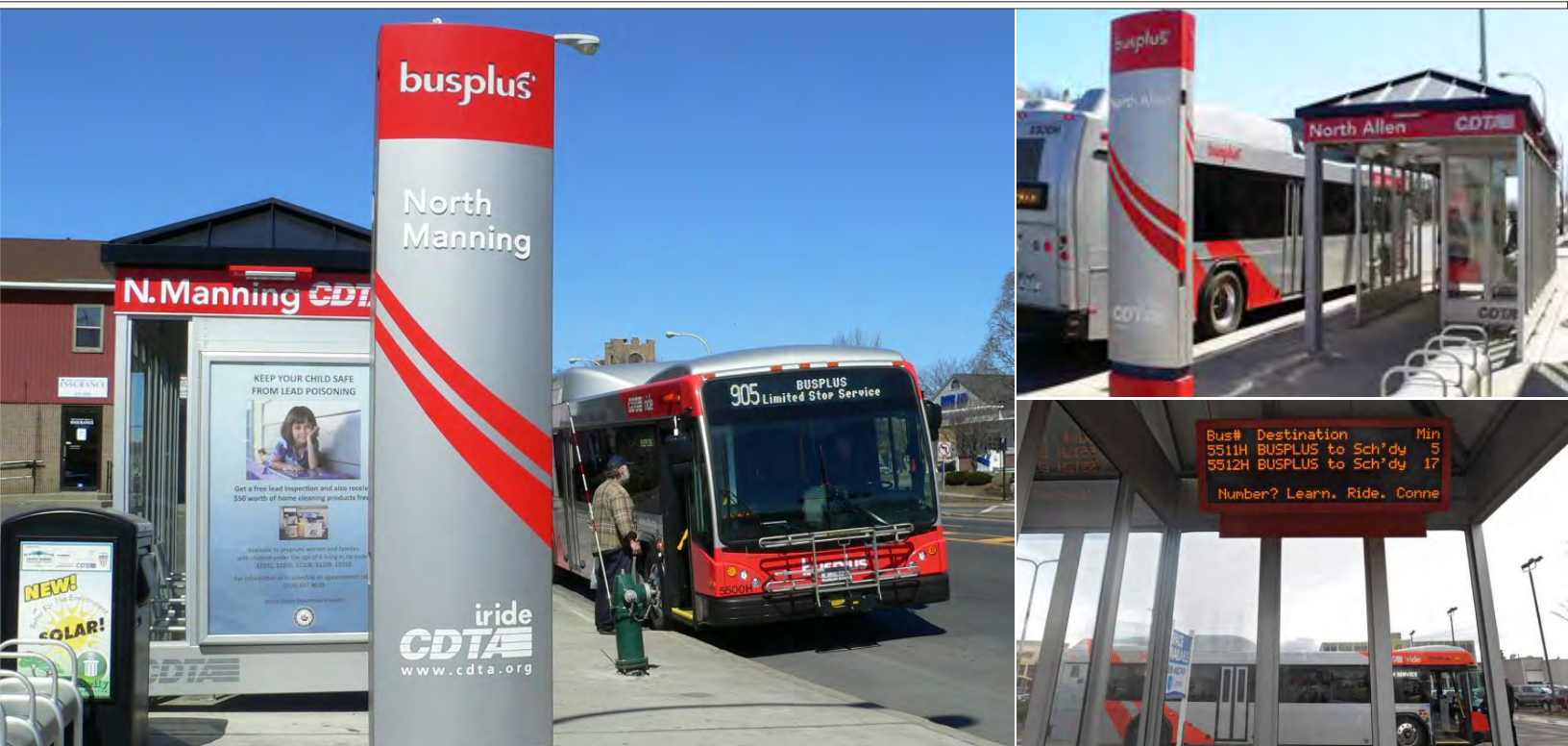
Figure 2.2.1: Enhanced Bus Stop in Albany, NY
