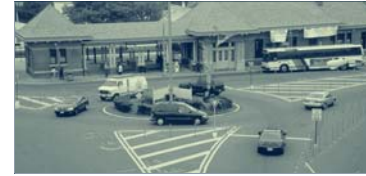
In Rutherford, a new roundabout was successfully tested by restriping the street and by using plastic bollards to direct traffic in new patterns.
