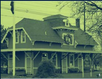
1 The Hilldale Train Station building and grounds have tremendous potential to serve as venues for community events, programs and information.
