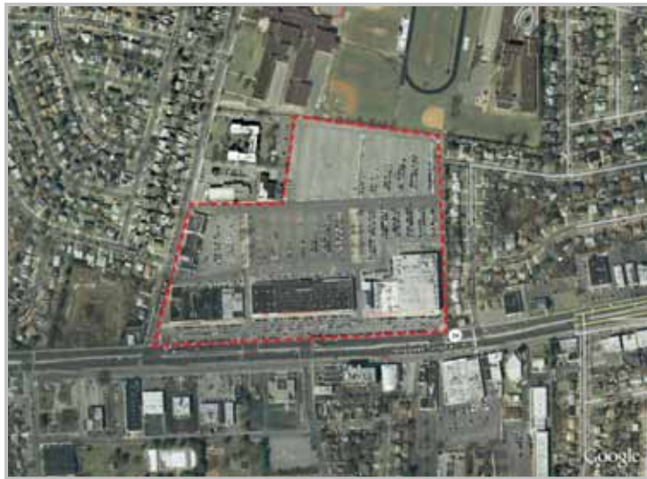
Figure 3-10 Community Shopping Center: Aerial Photograph
