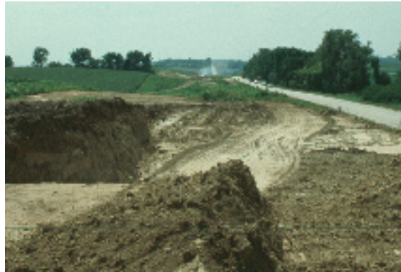
New Road Construction
