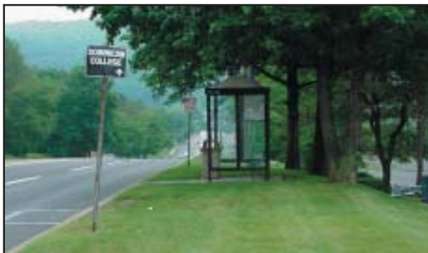
Sidewalks would improve the walkability of this area of Orangeburg
