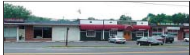
Existing conditions in a plaza on Route 303
