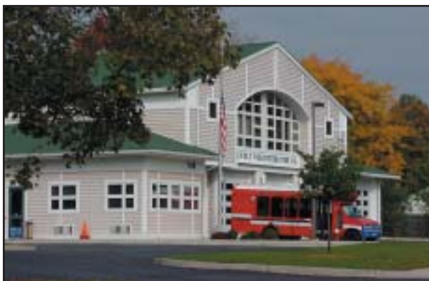
The new fire station in Blauvelt's hamlet center
