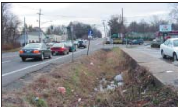
A drainage area along Route 303; increased protection and/or beautification should occur
