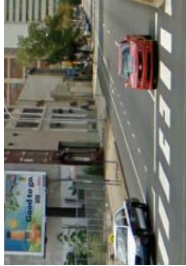
Wide vehicle travel lanes create additional impervious surface and may encourage higher vehicle speeds.
