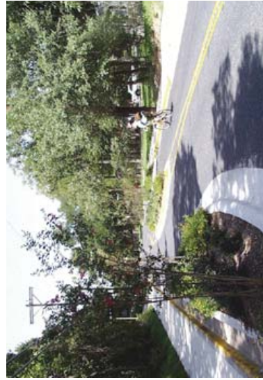
Chicanes are used for traffic calming and stormwater management, particularly near parks in Portland, OR. (streetsblog).
