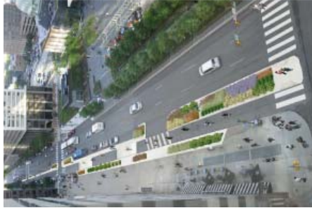
The above rendering of a proposed Center City Philadelphia Cycle track (Image courtesy of Center City District) shows how cycle tracks may be separated from adjacent travel lanes using parking lanes, raised pavement, planters, or other treatments.
