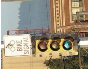
Bicycle signals should be accompanied by a "Bicycle Signal" sign to provide clarification for motorists and cyclists.
