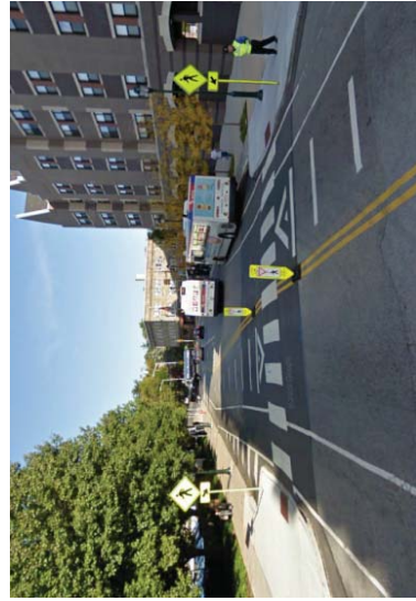
Raised crosswalks should be accompanied by signs and pavement markings to alert motorists of the crossing and pavement change. Detectable warnings should also be used for pedestrians. (54th St south of City Ave)
