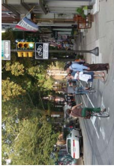
Buffered bike lanes (4.5.3) on Pine Street provide additional protection and comfort for cyclists.
