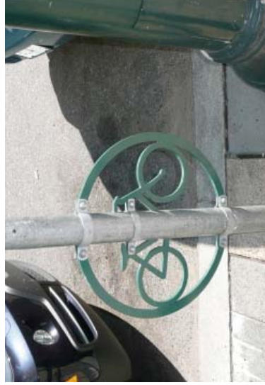
As individual parking meters are replaced with “smart meters”, meter poles may be repurposed as bicycle parking.
