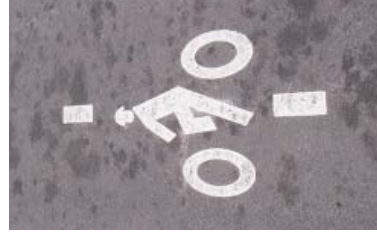
Bicycle detection should be provided at signalized intersections if the phase(s) serving bicycle movements is not set to recall each cycle. The "Bicycle Detector" pavement marking and sign (MUTCD 9C-7 and R10-22) should be used at intersections with in-pavement detectors.
