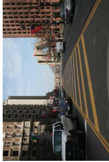
Painted medians provide some traffic calming benefits, but do not provide a protected refuge for pedestrians.
