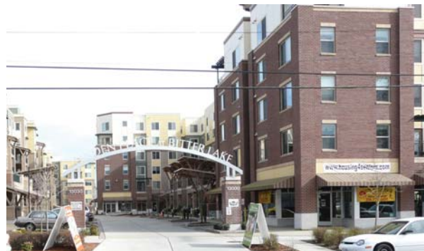
Build on the design precedent set by the Cambridge and New Haven, incorporating substantial brick and mixed finishes, strong detailing, modulation and ground floor shops like Seattle Mobile Espresso.
