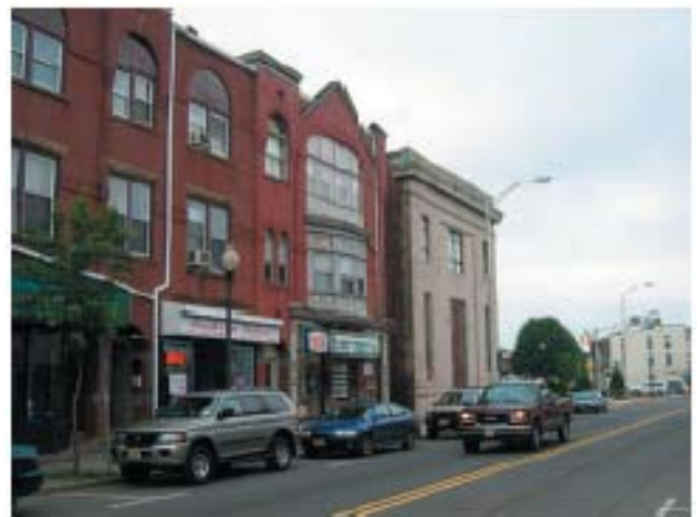
Historic buildings along Main Street in Bound Brook.
