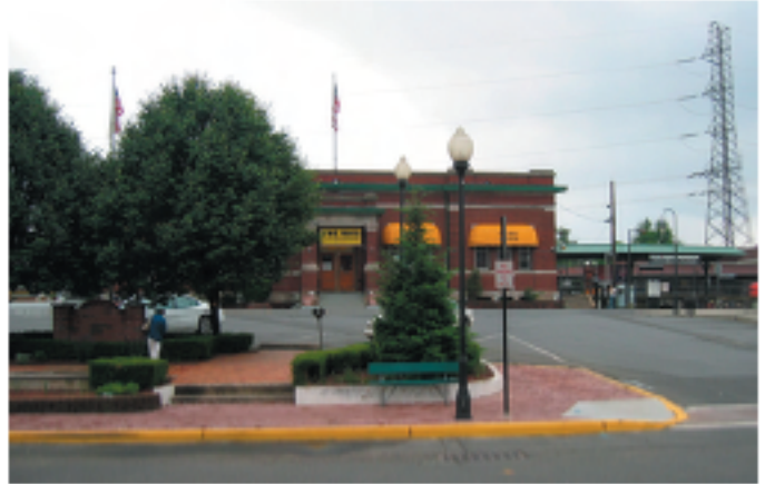
Drop-off area at Bound Brook Station.
