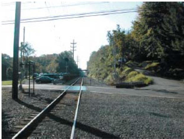
Existing North Branch Station.
