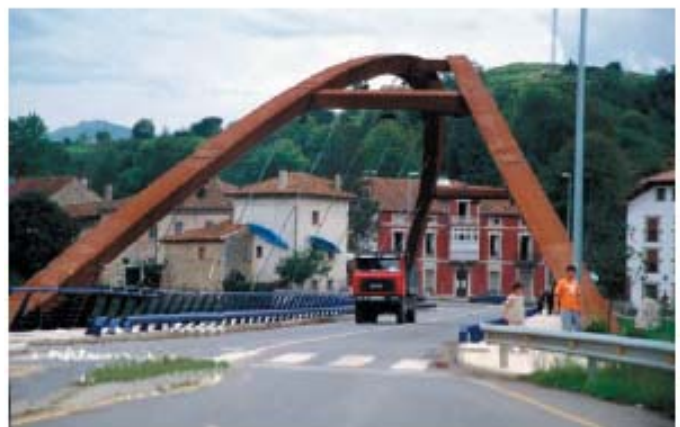
Example of a multi-use bridge.
