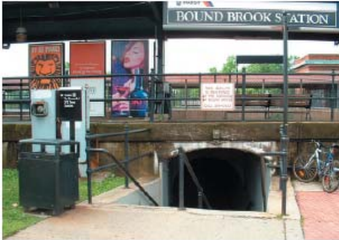
Pedestrian-underpass at Bound Brook Station.
